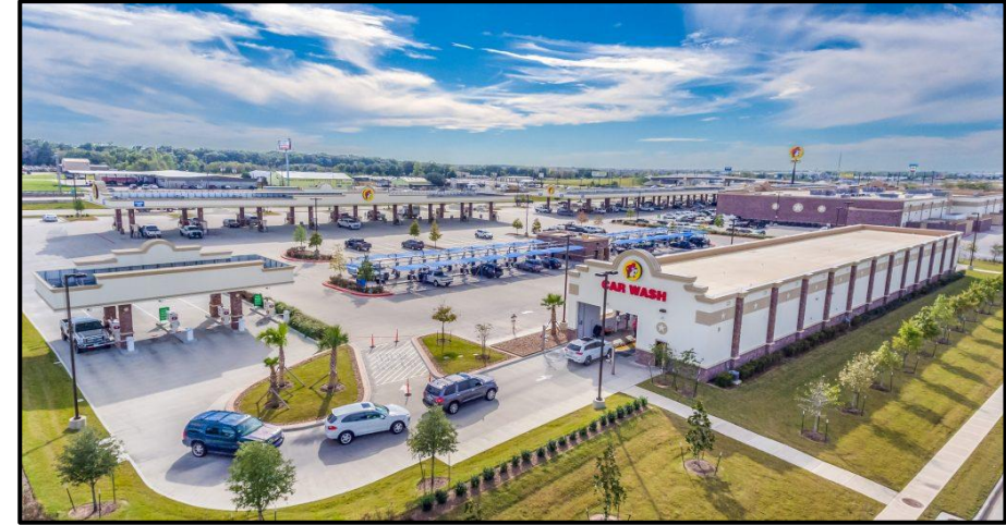
New 53,000 sq. foot BUC-EE'S opened August 2021, 8-minute drive from site
